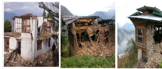
Figure 7a, 7b & 7c: Traditional house in Eastern Bhutan heavily damaged by 2009 earthquake. Photo: Rohit Jigyasu, Bank
